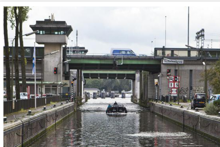
Figure 1. Example of a movable bridge (Schinkelbruggen, Amsterdam).
