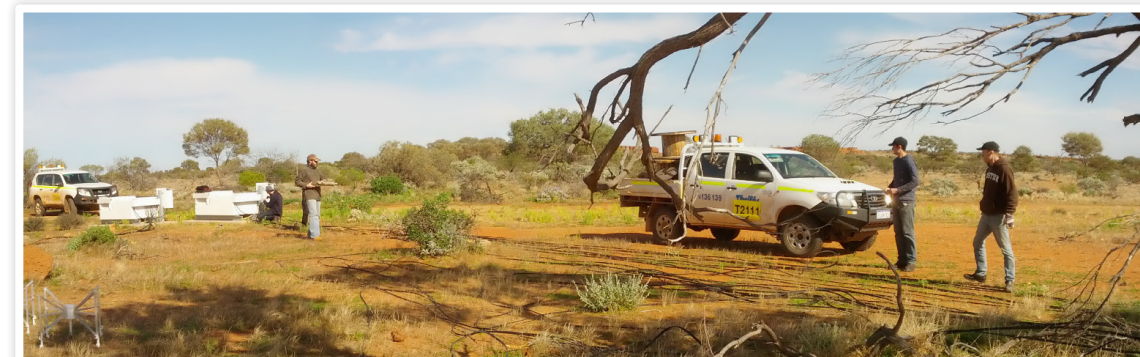
Figure 3: Laying cables in the unusual green desert.
